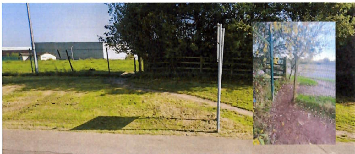
Figure 2: Existing break in the fence (inset) and unauthorised access on to the N40 at Garranedarragh
