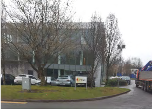
View of northern elevation
