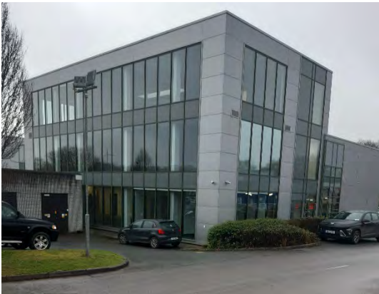
View of northern and western elevations
