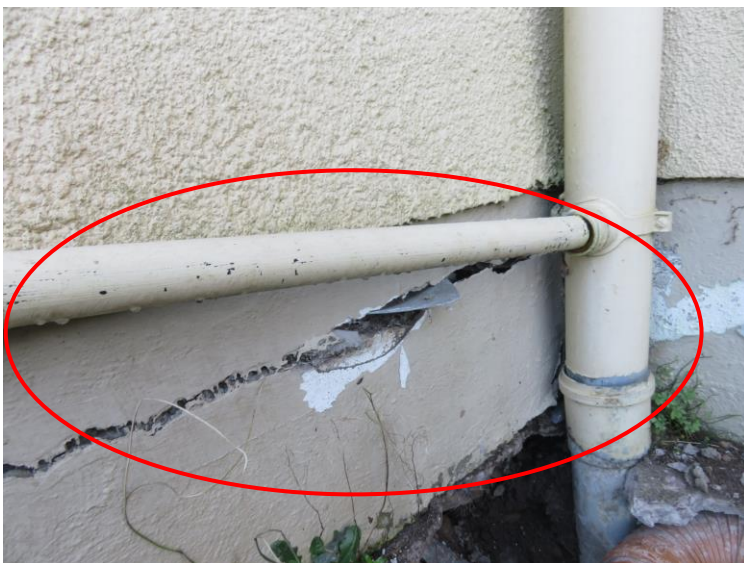
Side elevation of extension, large horizontal crack underneath existing window opening (approx. 20mm)
