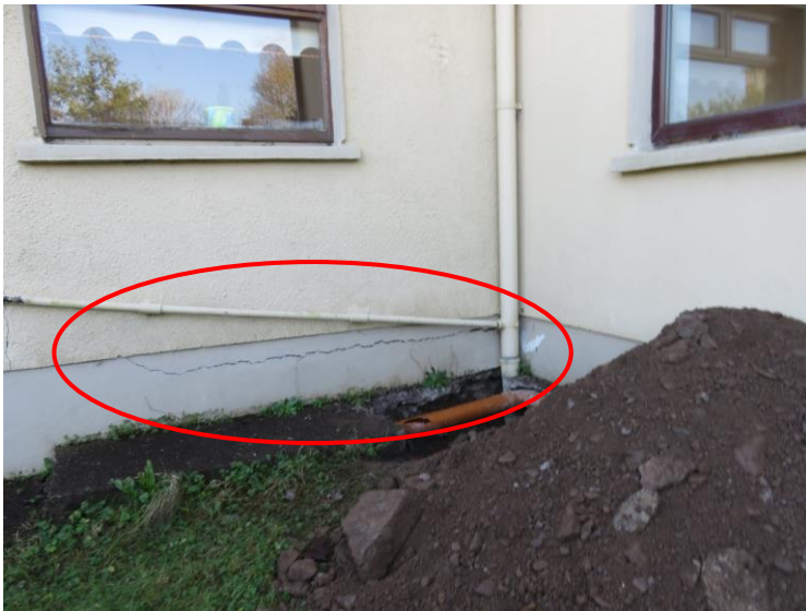
Side elevation of extension, large horizontal crack underneath existing window opening
