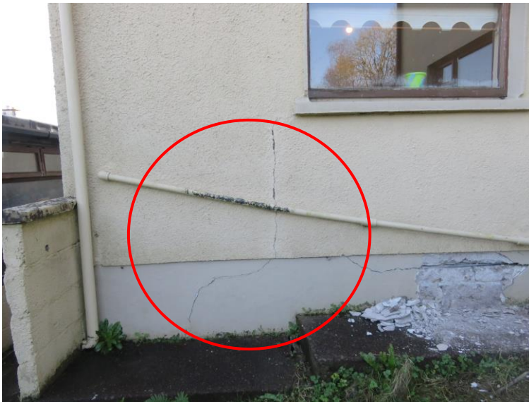
Side elevation of extension, vertical/diagonal cracking visible to left hand side of existing opening.
