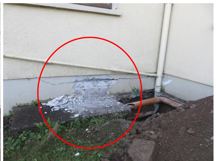
Excavation was carried out adjacent to the side wall of the extension to inspect foundations. The side wall of the extension is constructed on a slab visible externally (also the footpath). See photos above.
