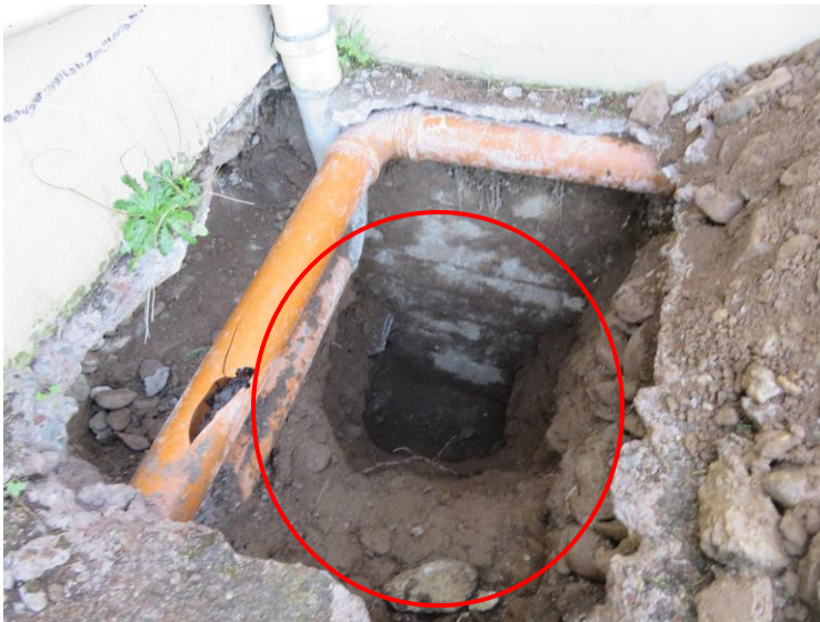
Foundation to main dwelling (circled) at depth (approx. 1.6m below finished floor level), extension side wall to the left hand side of photo.
