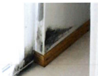
Lack of adequate ventilation can lead to mould growth due to condensation
