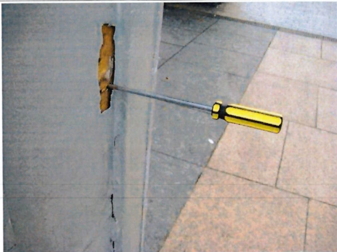
Photograph 22 View of timber decay and chipped paint to Column 2.
