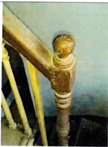
Newel post at half landing, showing a plain replacement baluster to left
