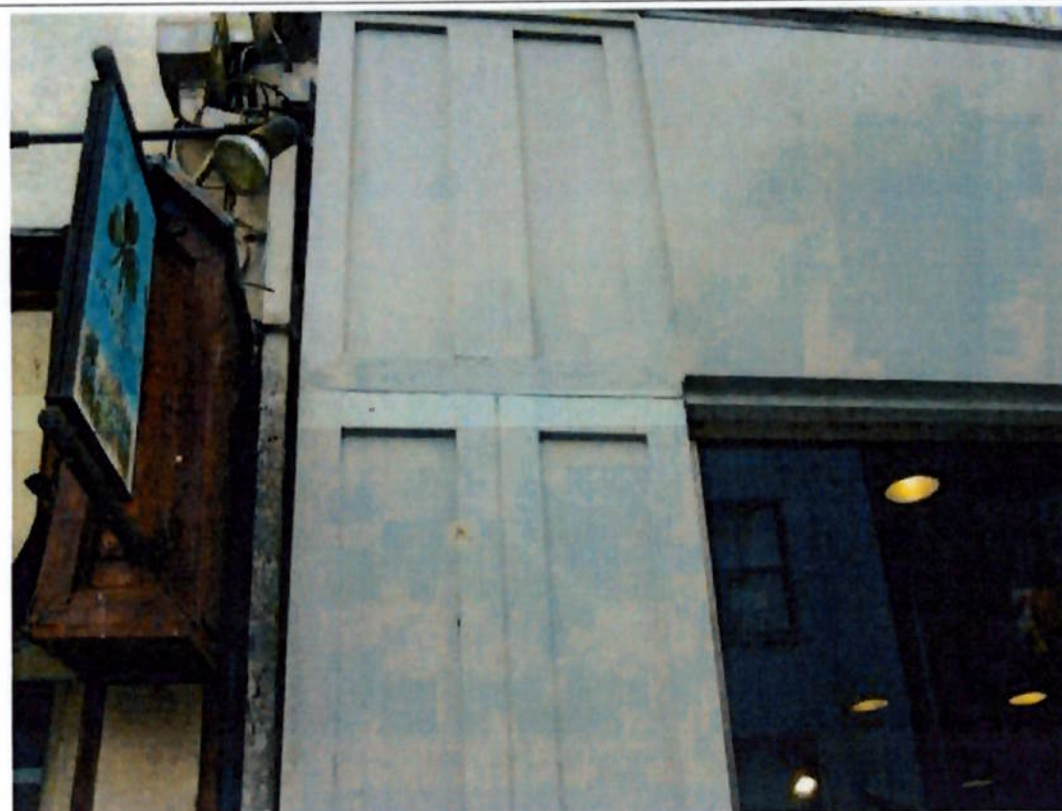
Photograph 27 General view of Column 1.
