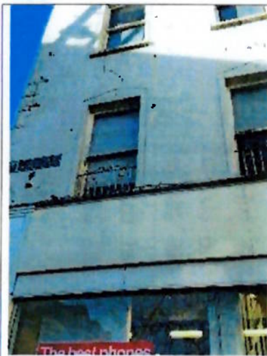
Western end of southern elevation, showing one of the cracks that needs to be stitched
