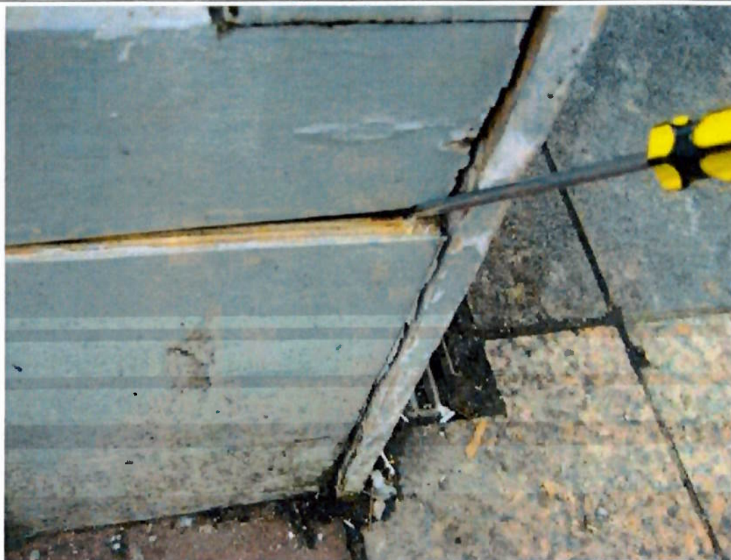
Photograph 23 View of screwdriver placed within a gap to the timber panels.
