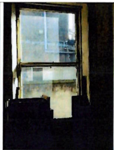
General view of one-over-one sash window
