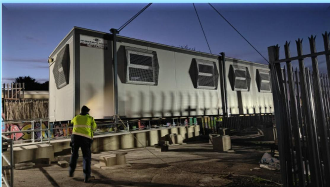
The new cabin was installed over the summer. IMAGE: Kabin Studio
