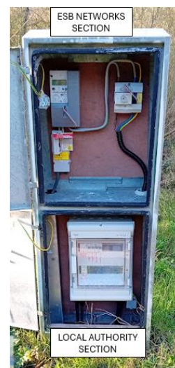
Location of DB in Metered Pillar
