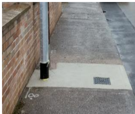
Access Chamber in Footpath
