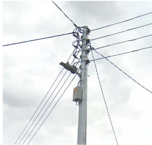
Under the ESB LV Conductor 0.3m Outreach Bracket
