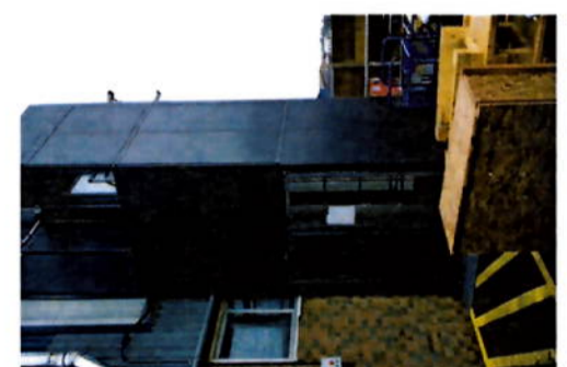
Example image of an external lift with ABS panel enclosure
