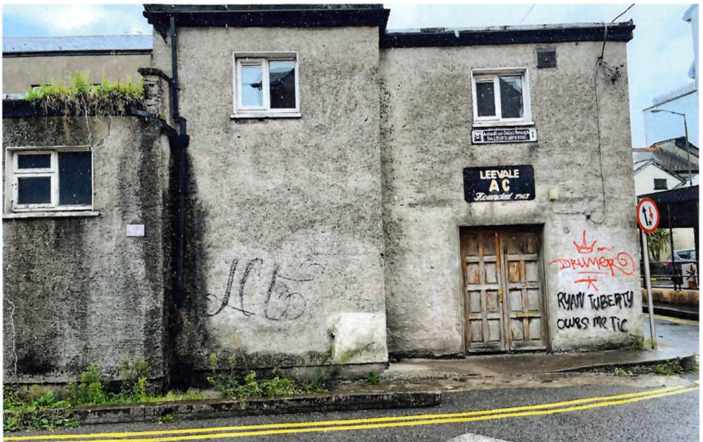
FIG 1 - Photo of premises prior to renovation works.
