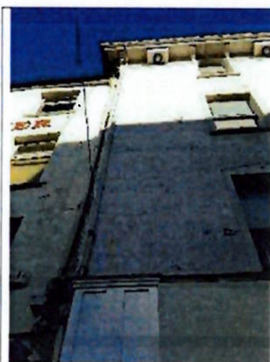
Western elevation showing horizontal cracks at first floor level where the elevation is bowing outwards
