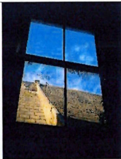
Two-over-two timber sliding sash window located in the northern elevation of the stairwell
