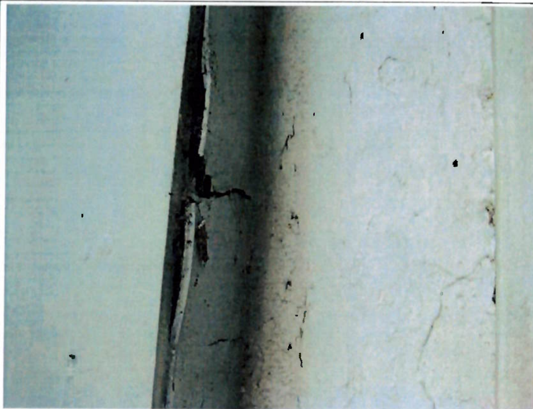
Photograph 7 View of chipped timber panel to Column 4.
