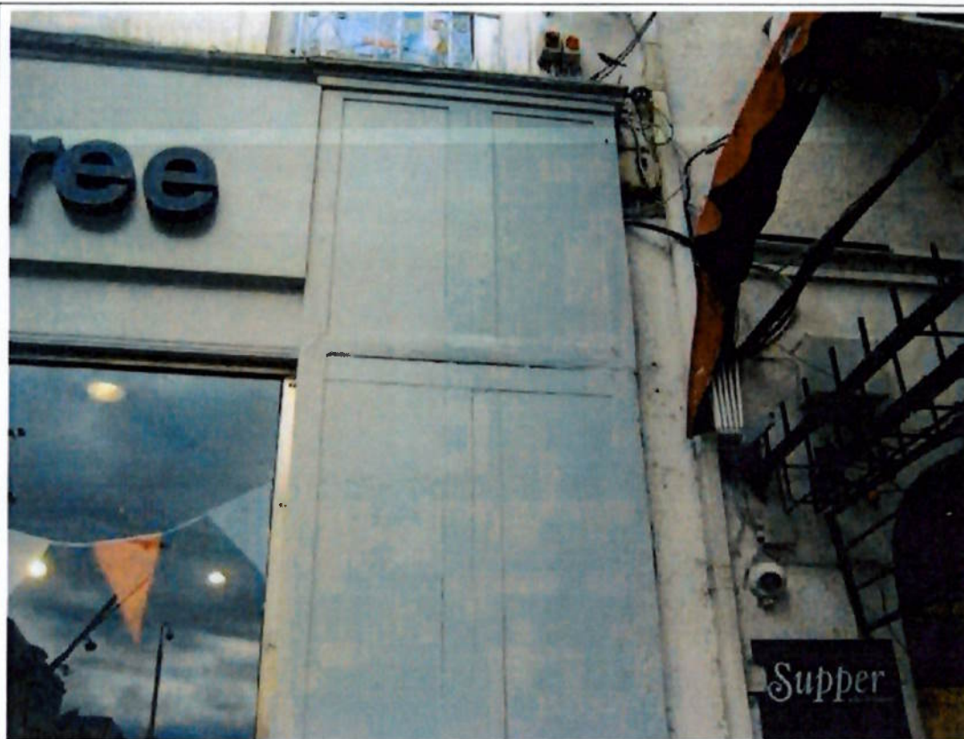
Photograph 3 View of timber decay and flaking paint to Column 4.
