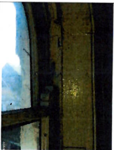
Round-headed one-over-one timber sliding sash window on the third floor.
