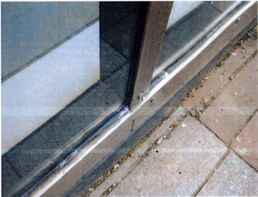
Photograph 25 View of perished mastic seal to the Side Elevation.
