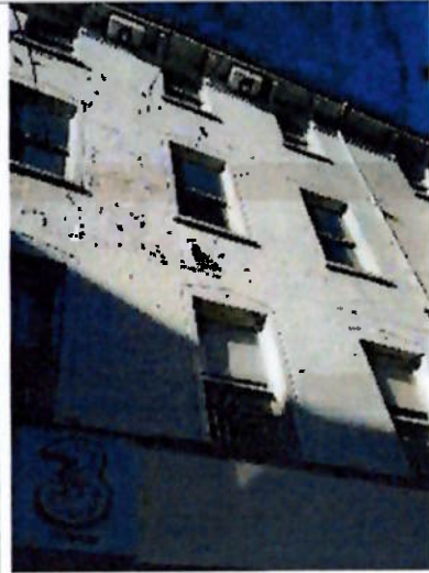
Southern elevation, showing cracked and peeling paint
