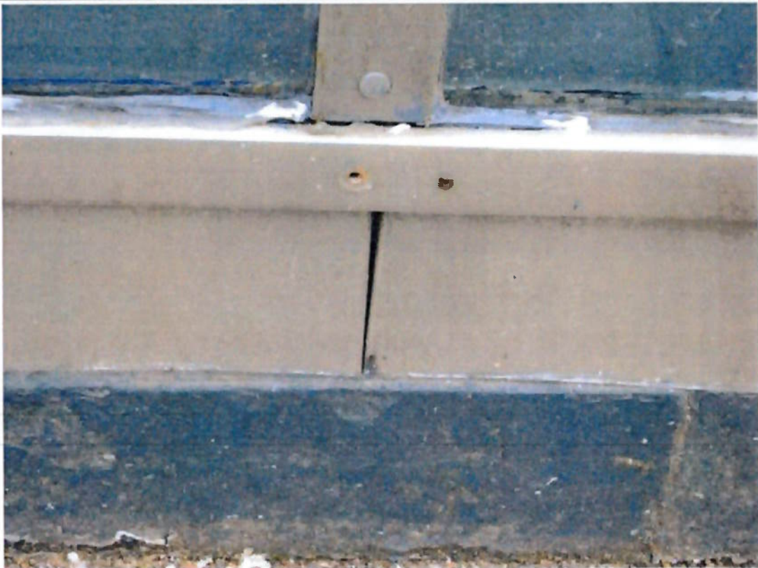
Photograph 26 View of missing screws and gap to the stainless steel plinth.
