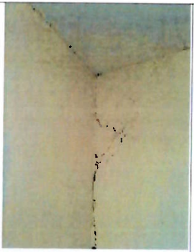
Serious cracking at the junction of the northern and western elevations of the second floor which needs to be addressed as a matter of urgency
