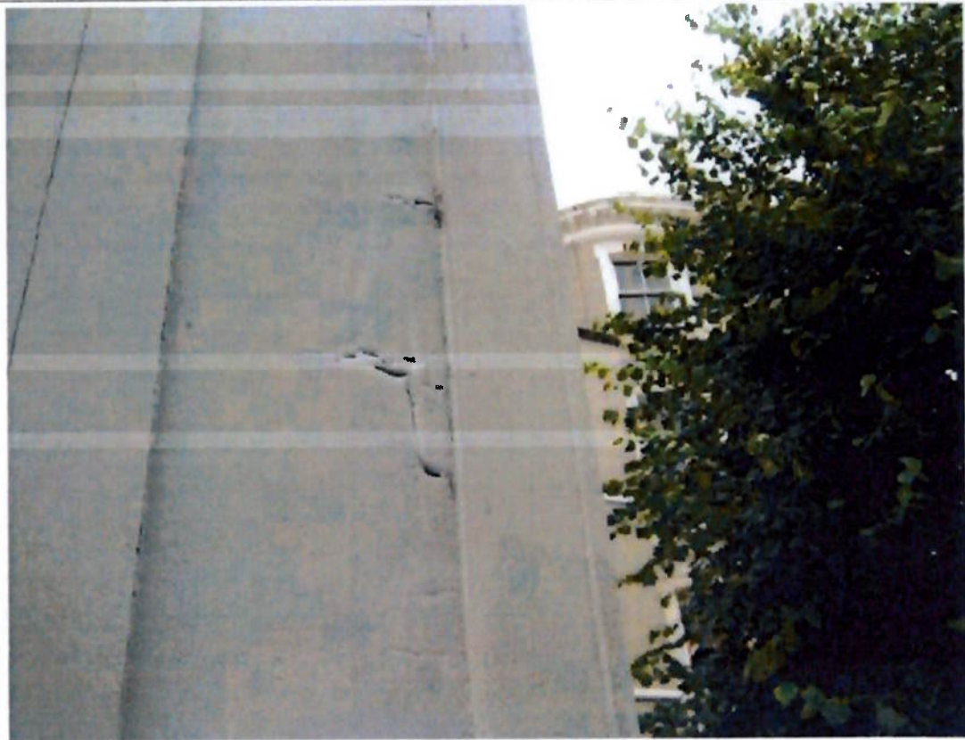
Photograph 21 View of blistering paint to Column 2.
