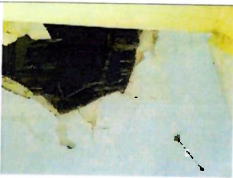
Hole in lath and plaster ceiling, where leaking water tank caused localised collapse
