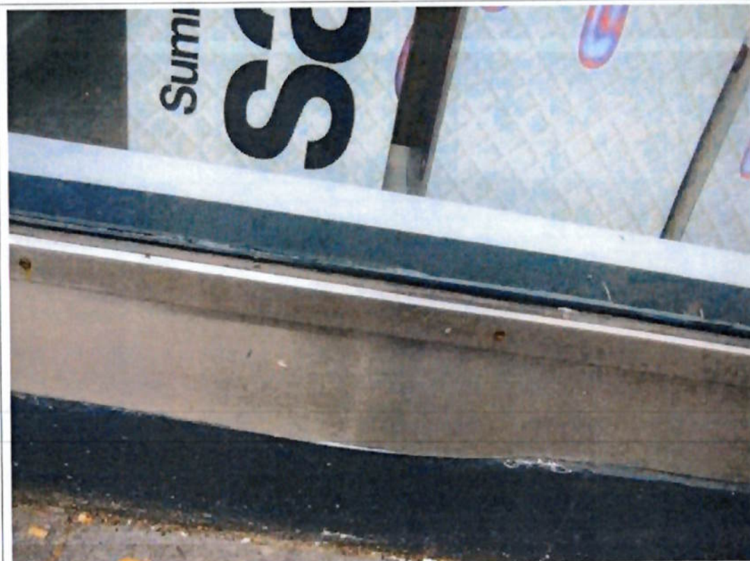
Photograph 14 View of deflected stainless steel plinth.
