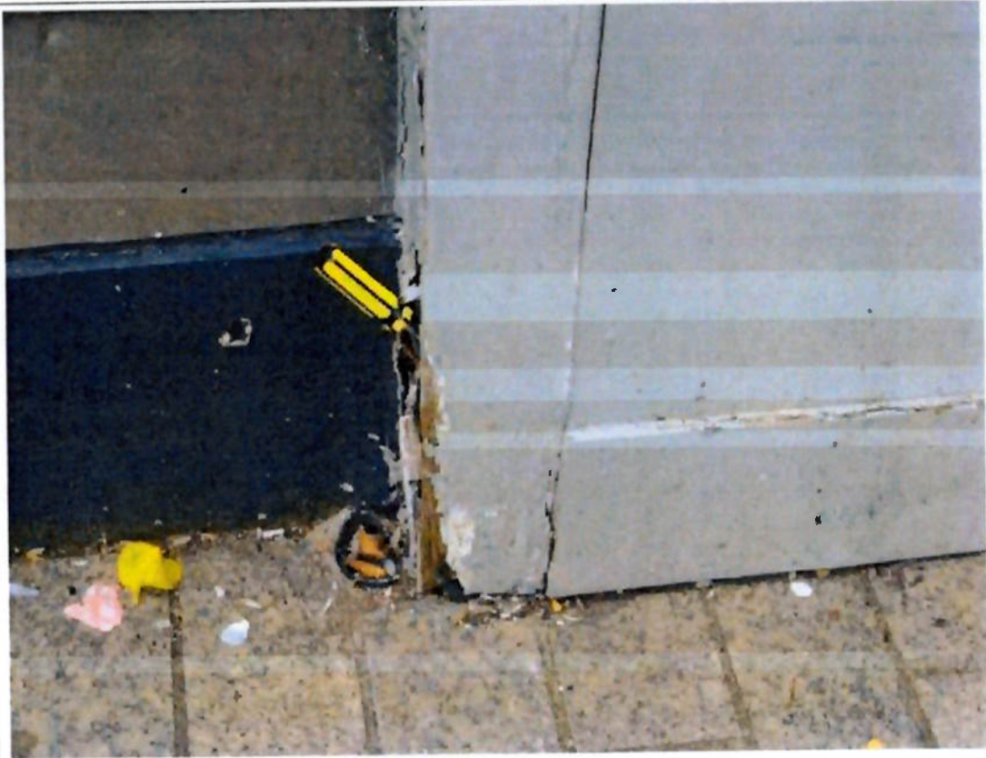
Photograph 5 View of chipped section to Column 4.
