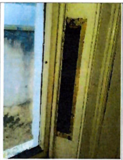
Sash boxes have been damaged in order to remove chords and pulleys on almost all windows
