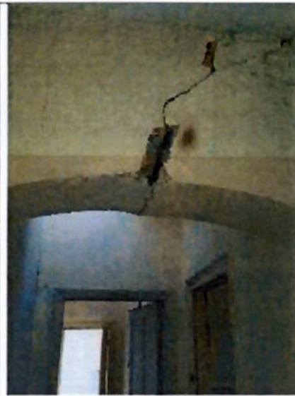
The northern side of the arch on the third floor also needs to be stitched
