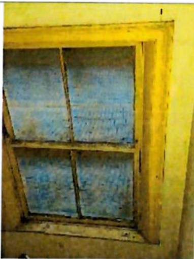
Two-over-two timber sliding sash window located in the northern elevation of the stairwell, showing architrave
