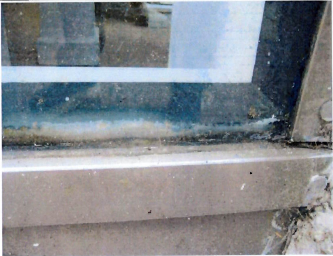
Photograph 9 View of perished mastic seal to the Front Elevation.
