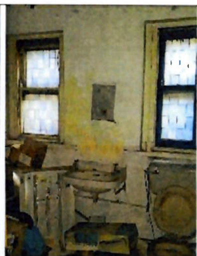
Mid-later twentieth century sanitary ware in second floor bathroom, showing sliding sashes with coloured decals
