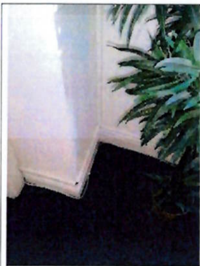
Late nineteenth century skirting boards survive on the first floor, with minimum intervention from cabling added later
