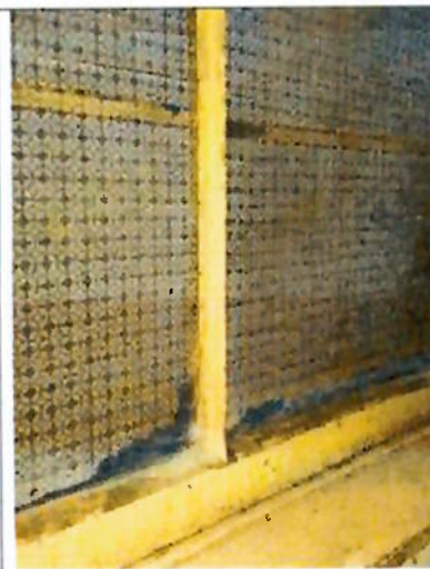
Two-over-two timber sliding sash window located in the northern elevation of the stairwell, which has been covered with opaque decals
