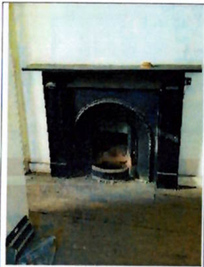
Standard cast iron fire surround dating to 1880s
