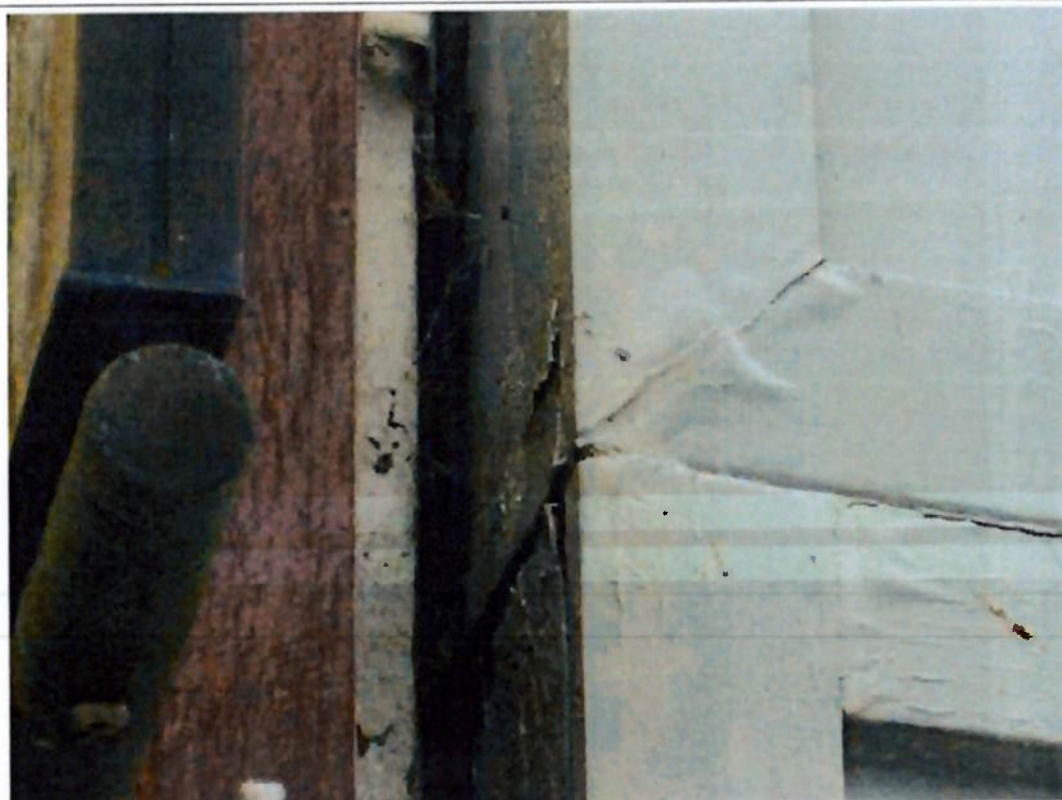
Photograph 28 View of blistering paint to Column 1.
