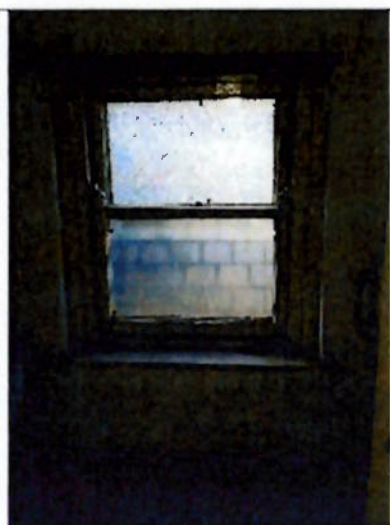
One-over-one timber sliding sash window in bathroom in northern elevation
