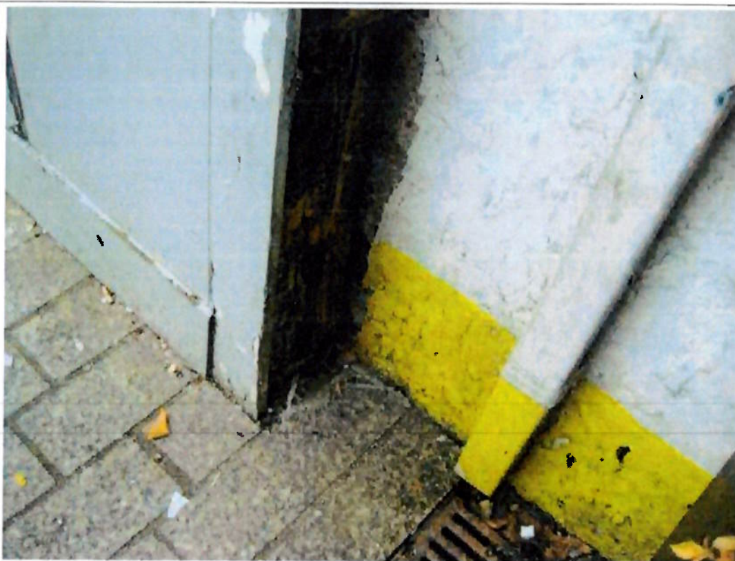
Photograph 8 View of missing timber panel to Column 4.
