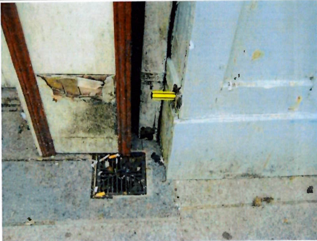
Photograph 31 View of screwdriver puncturing through decayed timber.
