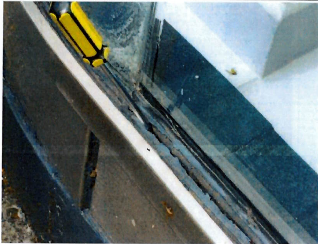
Photograph 11 View of screwdriver placed within a large gap to the mastic seal.
