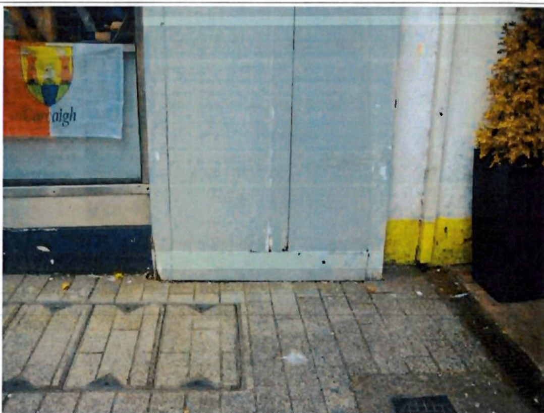
Photograph 4 View of timber decay and chipped sections to Column 4.
