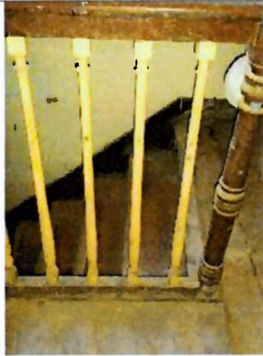
Four surviving Georgian balusters on the second floor landing, representing the earlier phase in the buildings development
