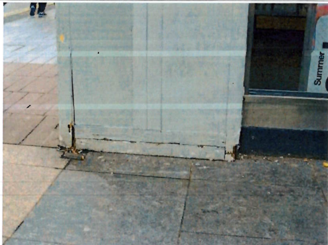
Photograph 16 View of timber decay and chipped sections to Column 3.
