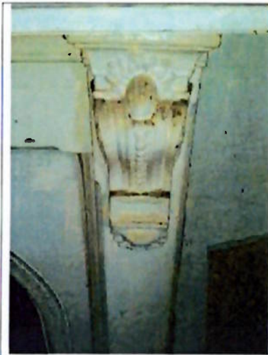
Detail of cast iron console bracket supporting mantel piece
