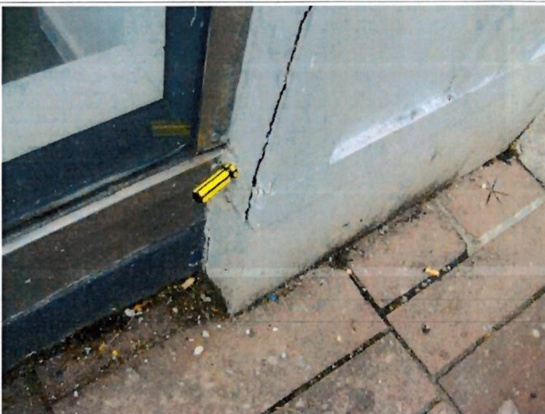
Photograph 24 View of screwdriver puncturing through decayed timber.
