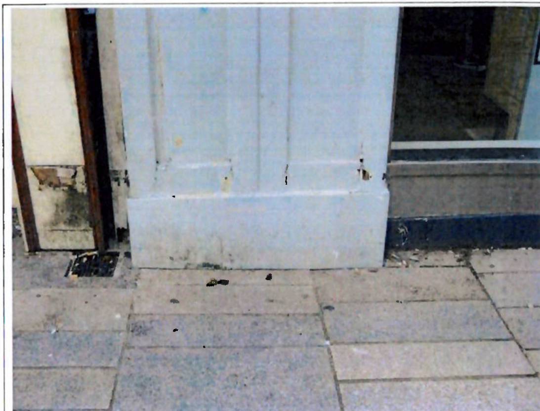
Photograph 29 View of chipped paint and heavy soiling to the base of Column 1.
