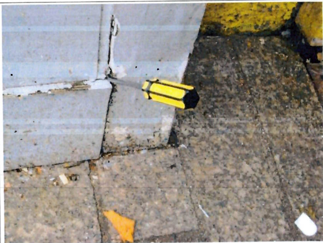
Photograph 6 View of screwdriver puncturing through decayed timber.
