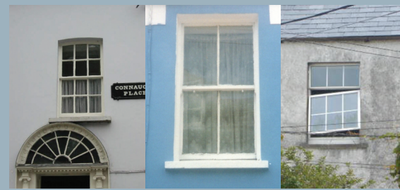
Well maintained original sash windows
