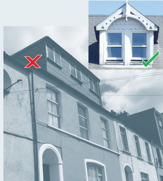
Example of an inappropriate box dormer
