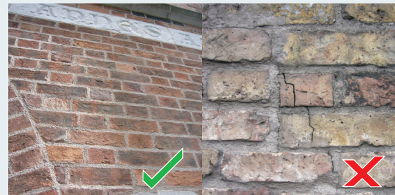
Lime mortar pointing
