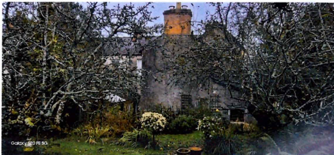
View of existing from rear
