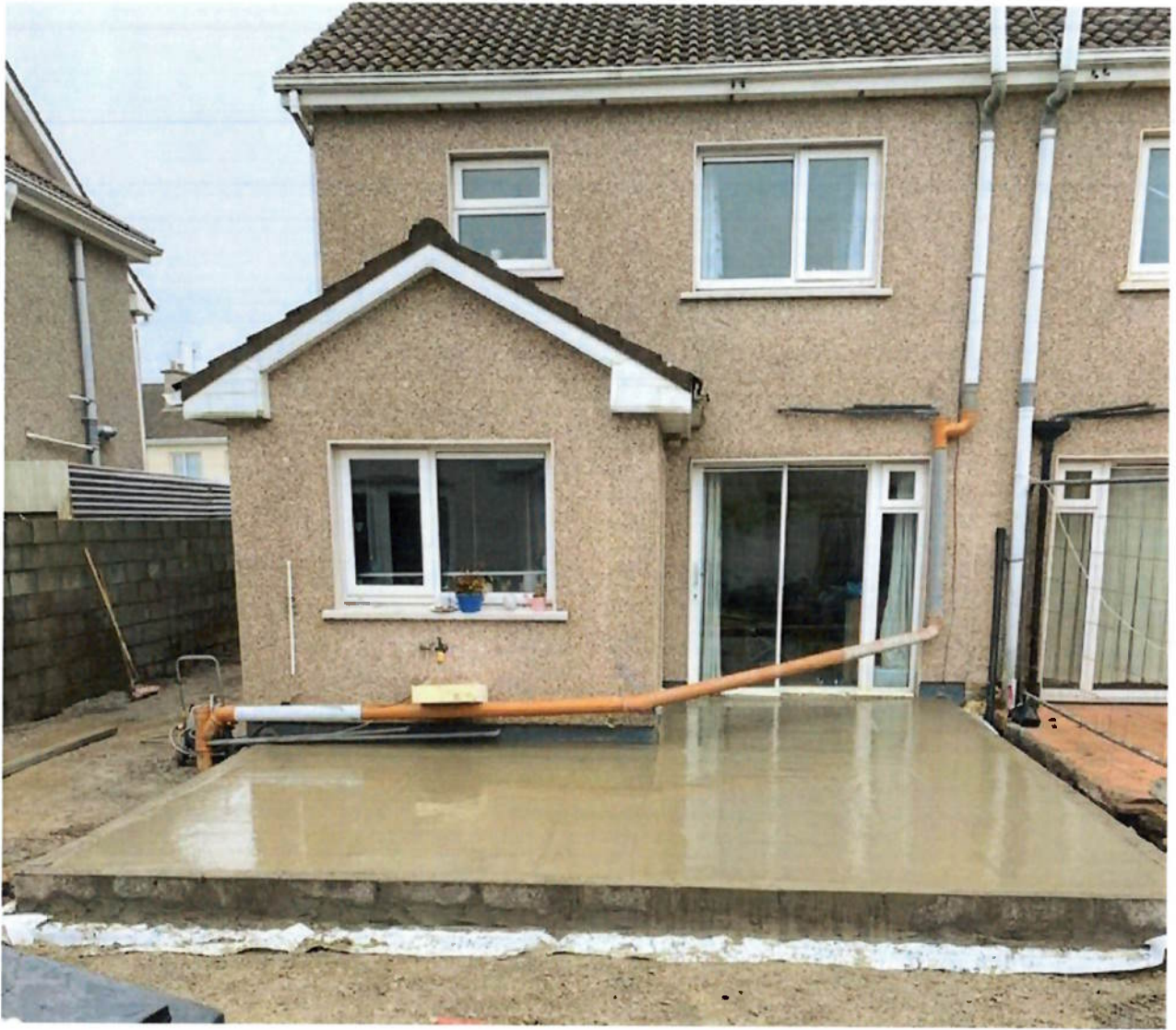
Image : External view of rear extension during construction stage
