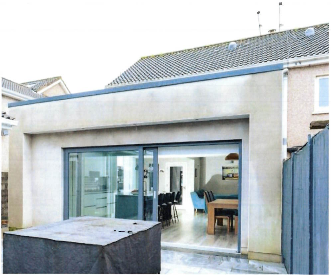
Image 1: External view of rear extension
