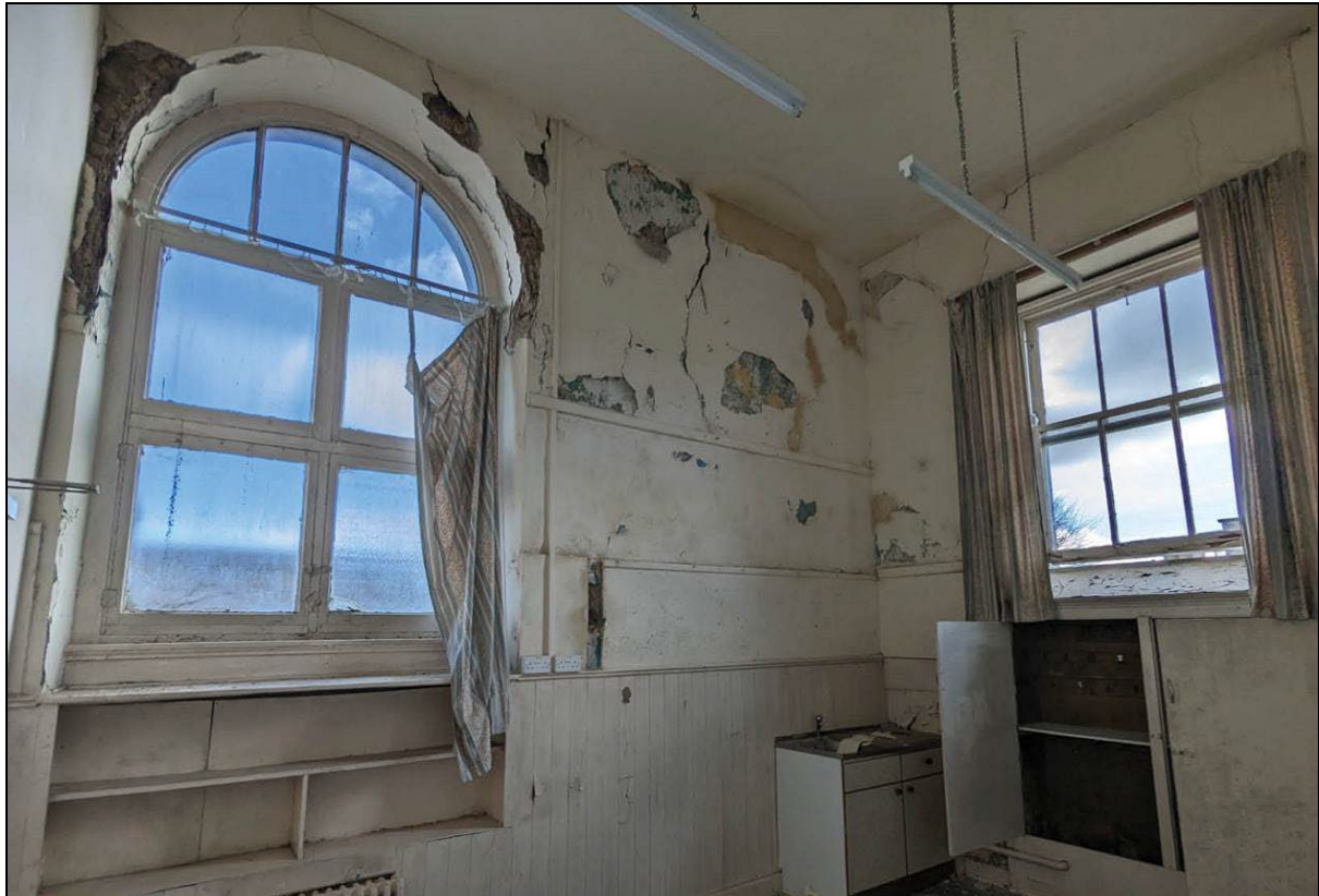
Room F11 looking SE.
