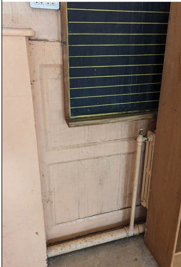
Detail of panneling to room G04
