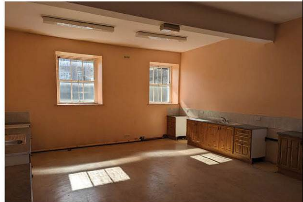
Room G04 looking SW showing windows.
