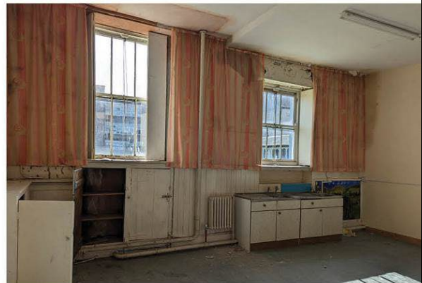
Windows to south of room G06.
