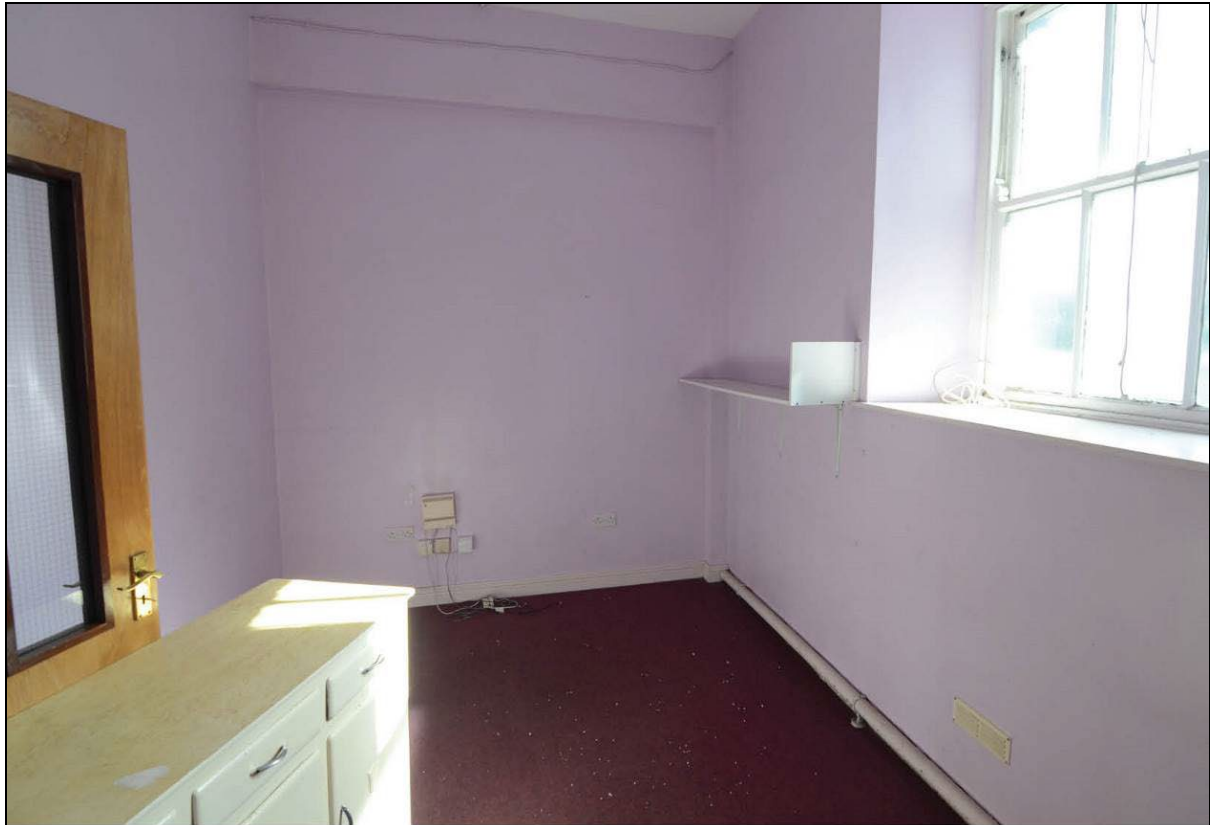
Room G03 looking SE.
