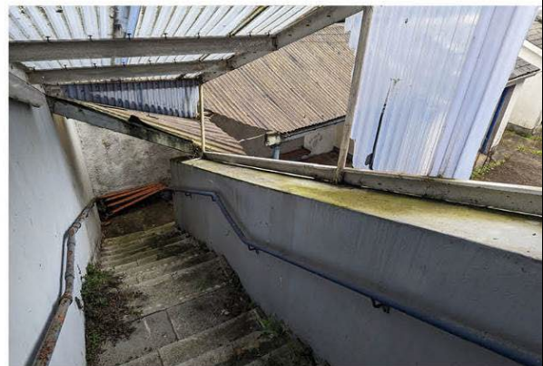
Western steps looking down towards yard.
