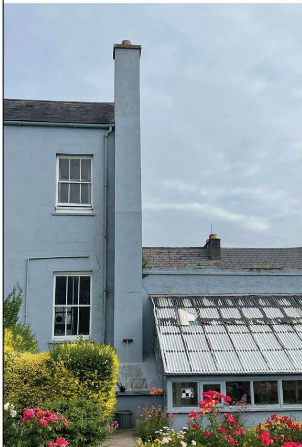
South elevation at east end showing chimney and greenhouse.
