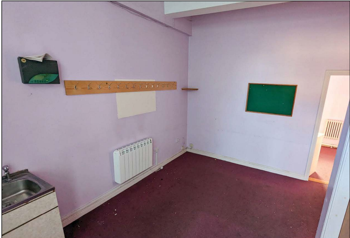
Room G01 looking SE.
