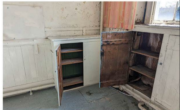
Panelling and cupboards in room G06
