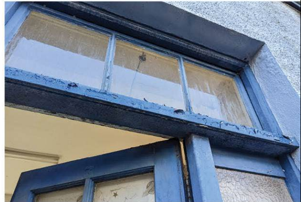
Detail of door to room G05.
