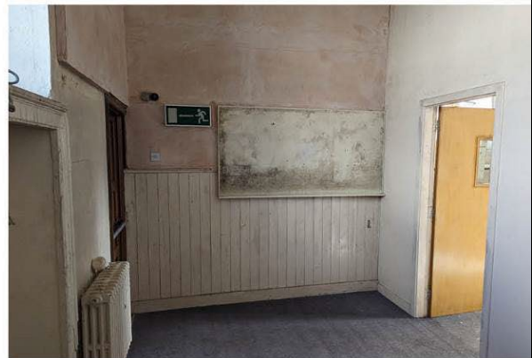
Room F09 looking east.
