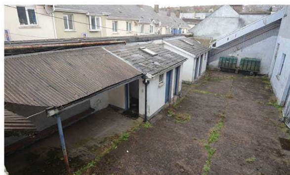
View of yard looking east showing toilet blocks and shelters.
