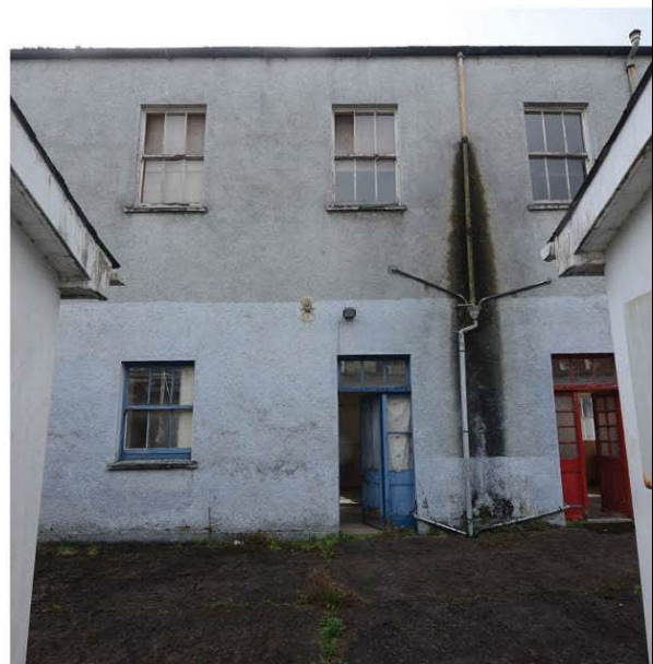
View of east elevation between flanking toilet blocks.
