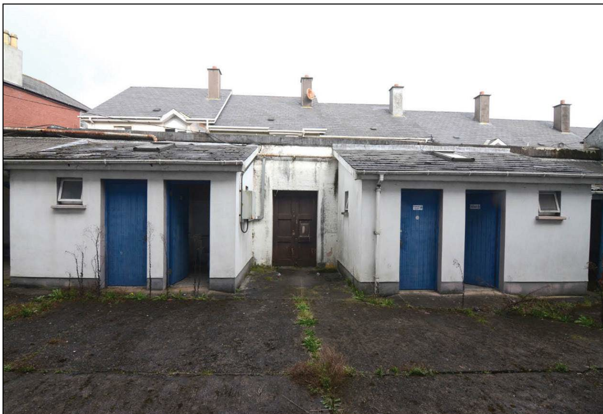
Toilet blocks to north of yard.
