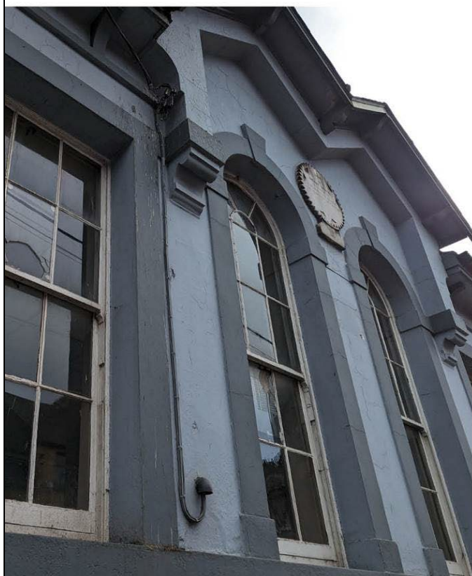
Infant school building on Gerald Griffin Street.
