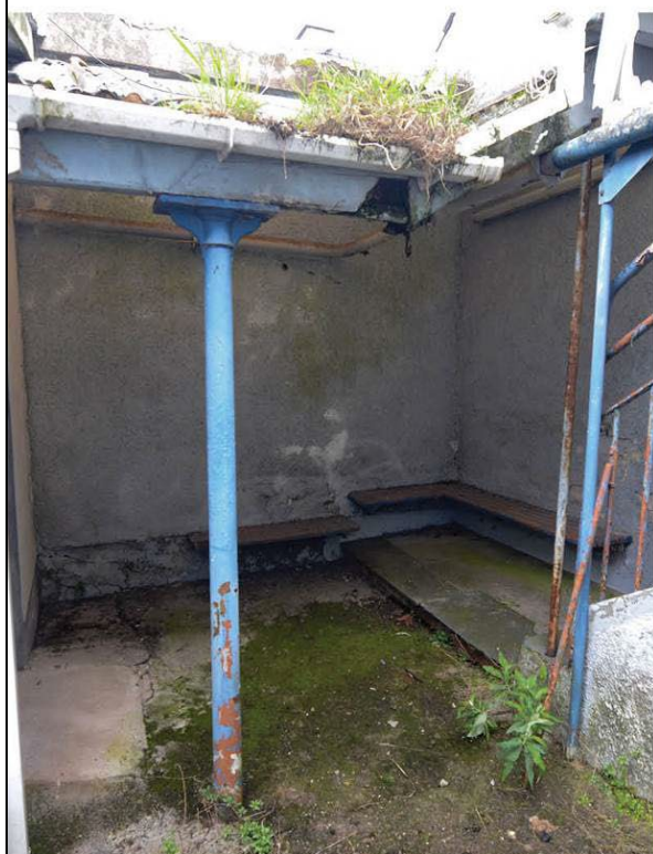
Shelter at east of yard.
