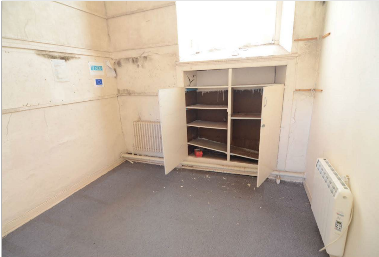
Room F06 looking south.
