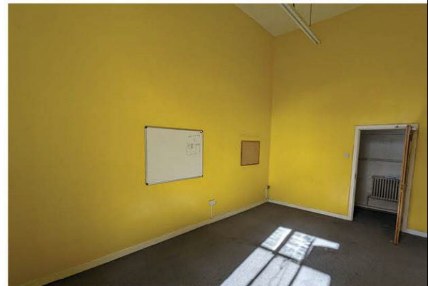
Room F10 looking NW.
