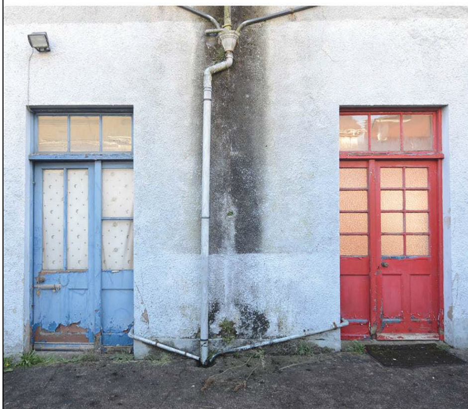
Detail of doors to rooms G04 and G05.
