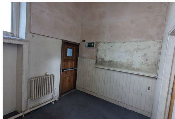
Room F09 showing door to eastern external steps.
