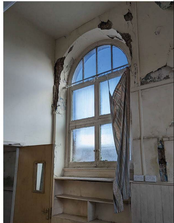
Window to west of room F11.
