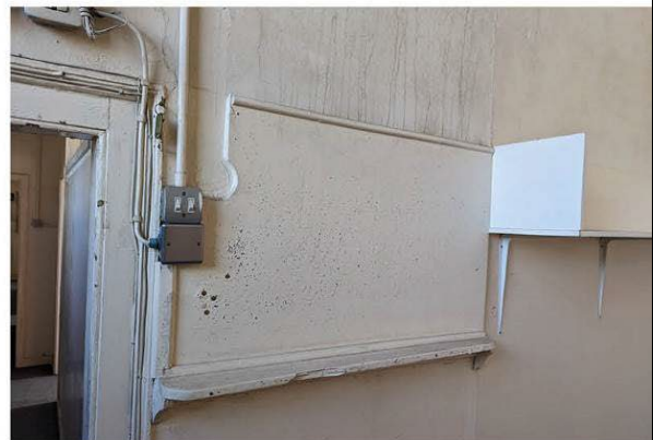
Detail showing architrave and various timber fittings in Room F03
