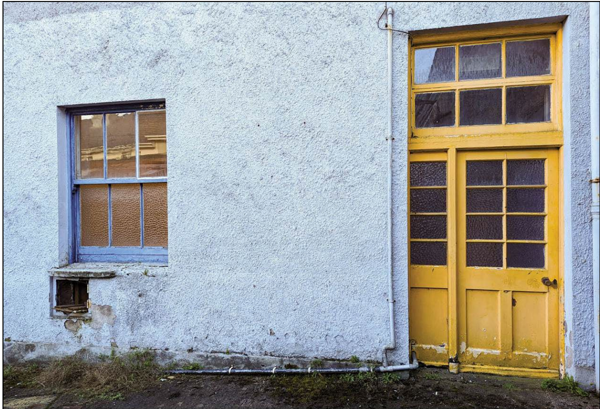
Door to room G01 and window to G04.
