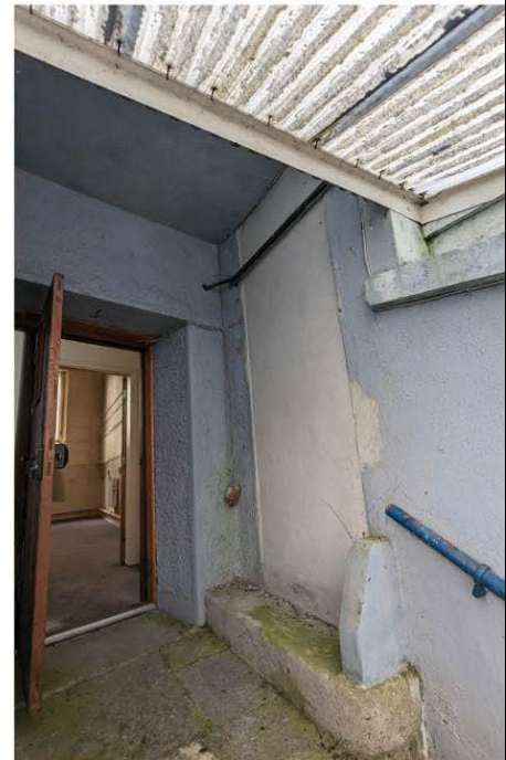
Top landing of western steps showing blocked doorway on right.
