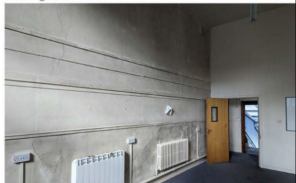
Room F02 showing door to F01 and external steps beyond.
