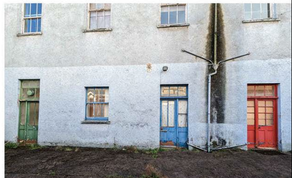
View of north elevation showing the doors.
