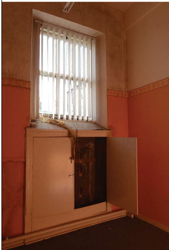
Room F03 looking south.
