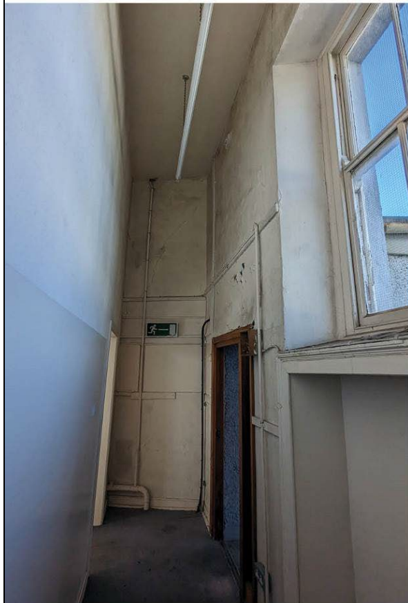
Room F01 looking west.
