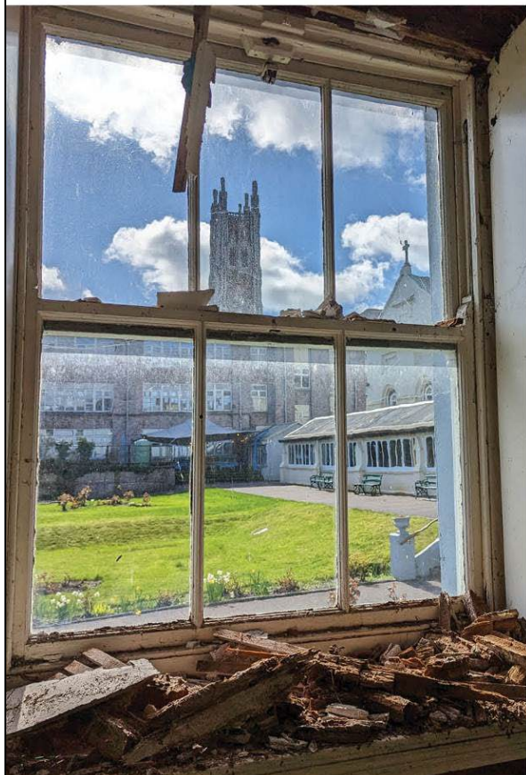
Window to south wall G05 showing detritus from collapsed lintel and view of garden beyond.
