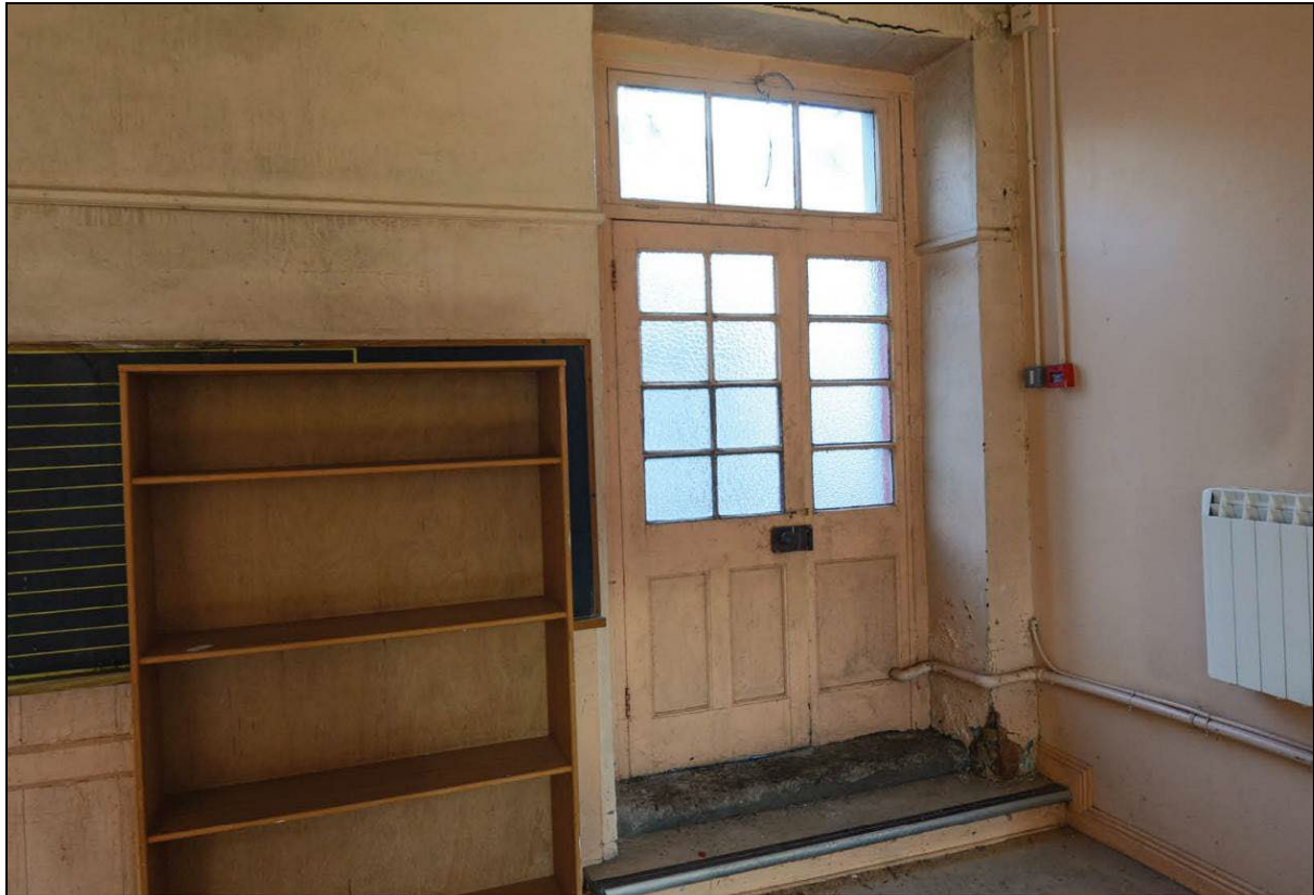
Room G04 looking NE.
