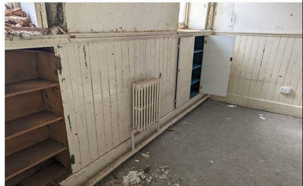
Pannelling and cupboards in room G05
