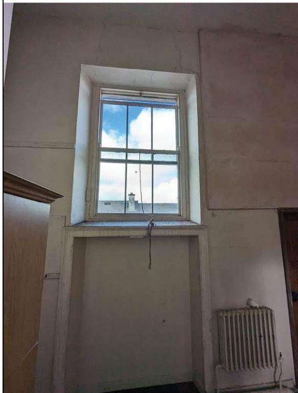
Window to north of room F09.
