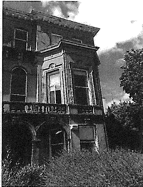
Photo 13 – South East Corner
