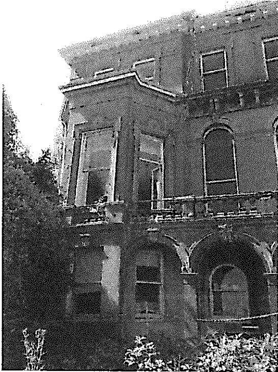
Photo 12 – South West Corner
