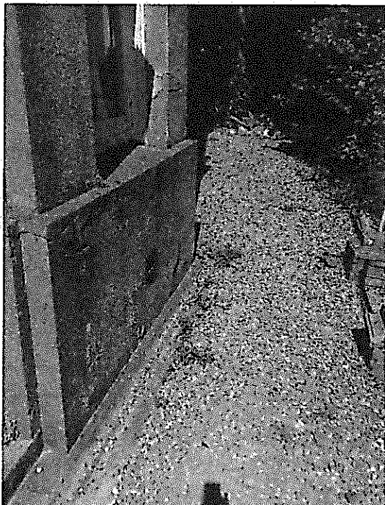
Photo 15 – Surface Drain and Gravel Path
